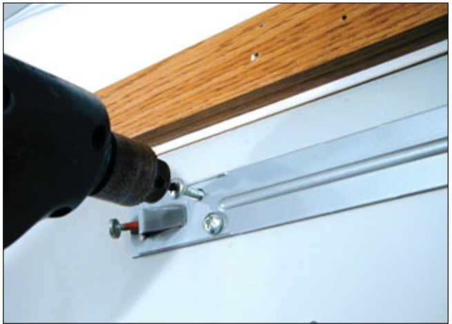
7. For metal doors, self-tapping screws are provided.
